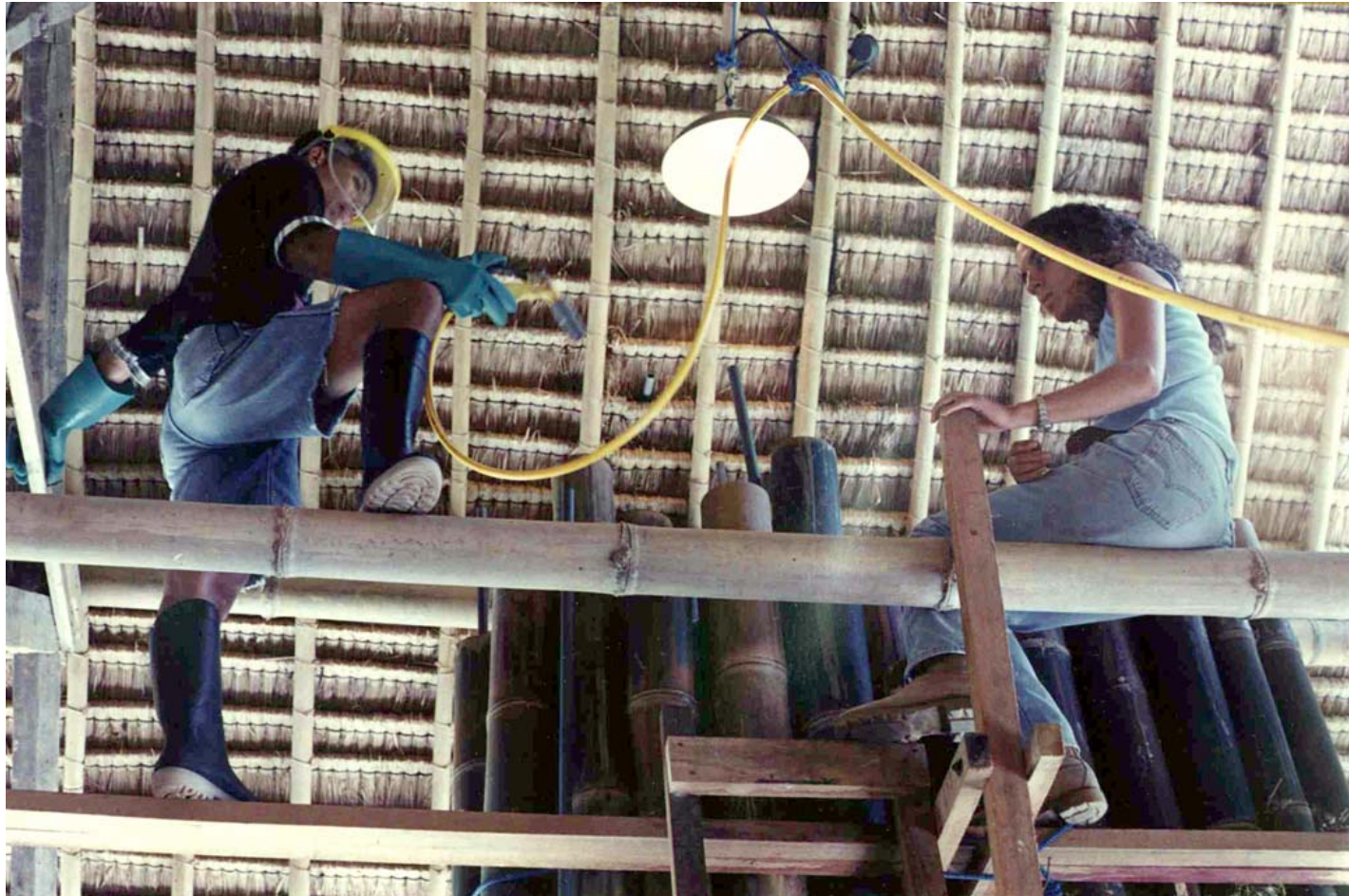
Filling the preservative into the lumina with their disrupted nodal walls, except the last node, to form a container, Thailand
