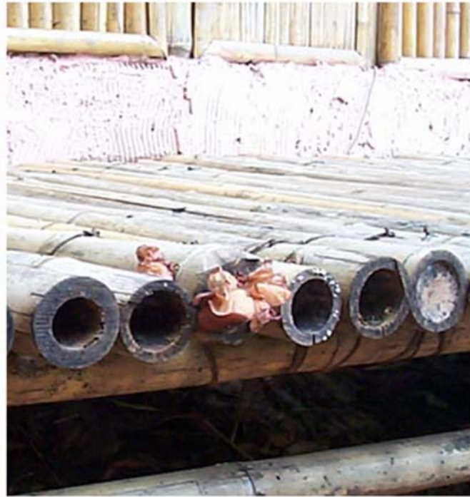
A newly built bamboo hotel is soon infested by fungi for degradation
