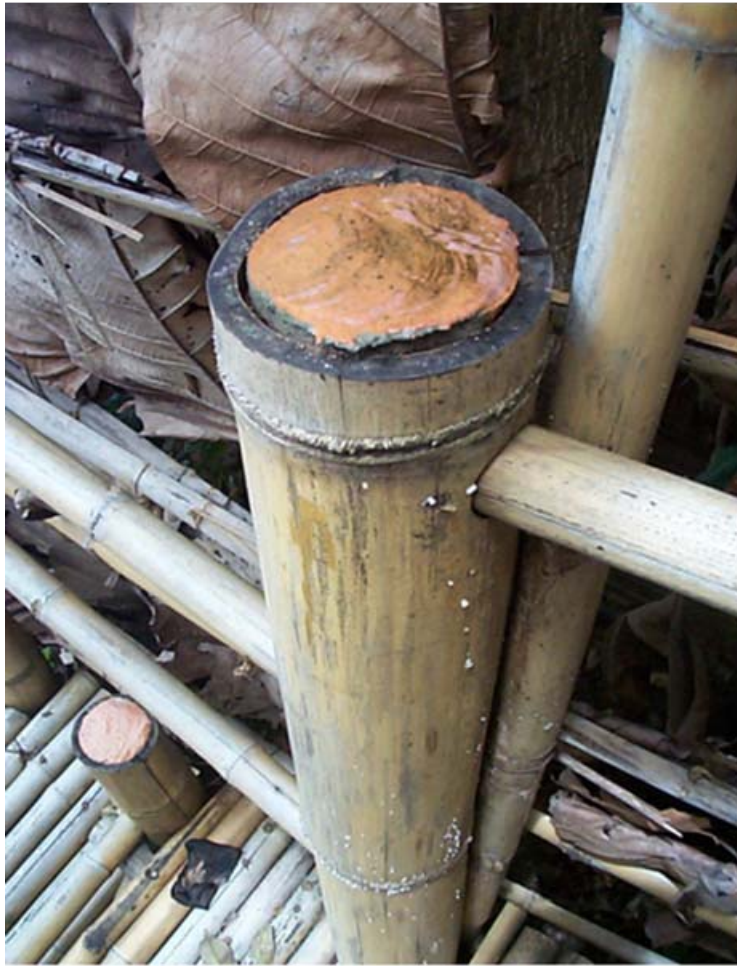
A newly built bamboo hotel is soon infested by fungi for degradation
