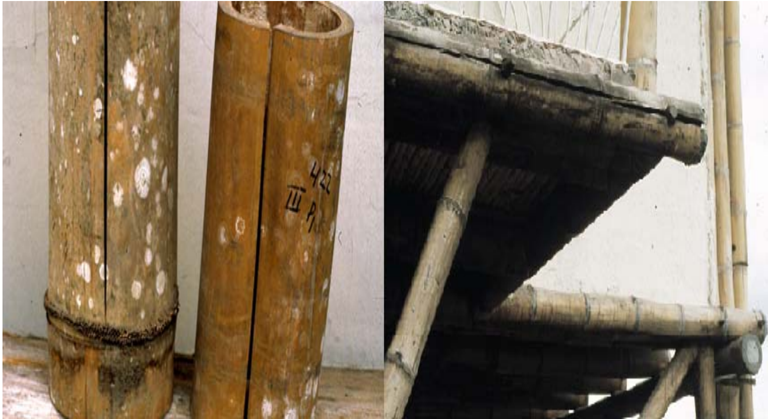
Construction failures due to weathering and splitting
