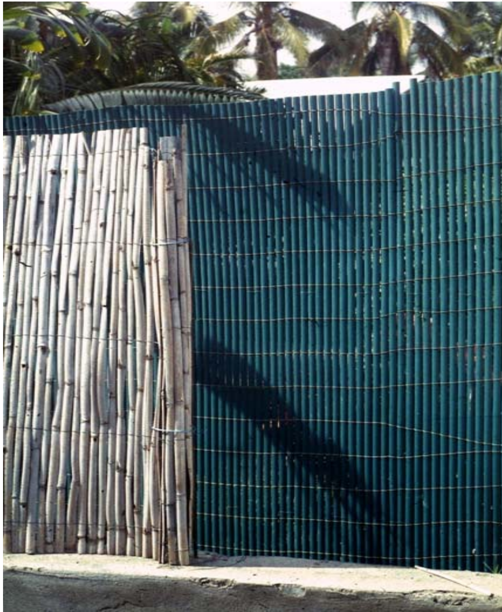
Walls, left from local bamboo with limited lifetime, right imported from China and quit durable
