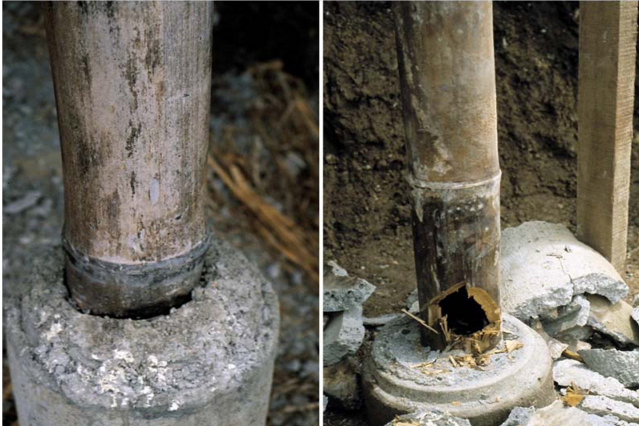
Culm embedded by cement causes shrinkage, with water collection causing fungal decay
